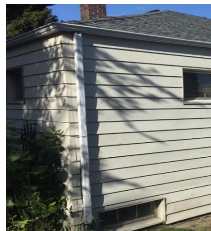
Straight Downspout Photo Credit: DZ/DG, 2018)
