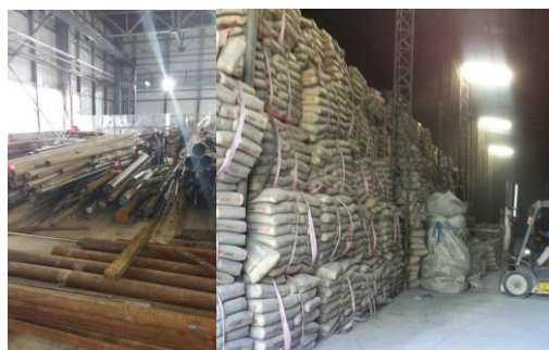
Figure4. Metal and Cement Storage
