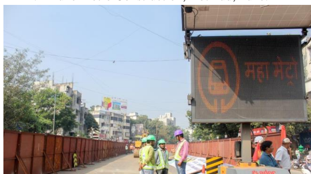
Figure 1 : Pune metro construction site
