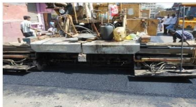
Figure 2 : : Unchecked asphalt paver machine
